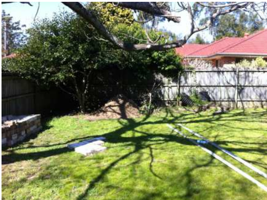
Figure 1.: Friday morning 9:52am – feeling positive – the build is underway!
