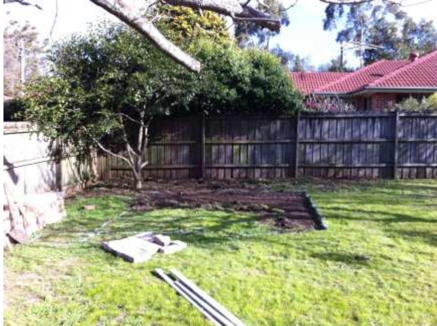
Figure 8.: Friday afternoon 3:19pm – digging for the floor finally started
