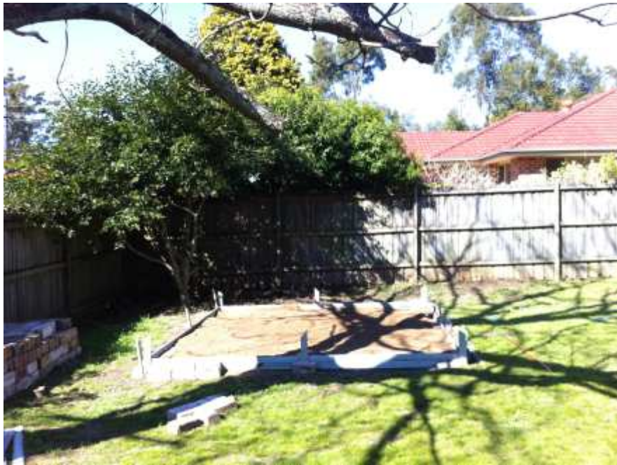
Figure 17.: Sunday morning 9:29am – sand spread, ready to level
