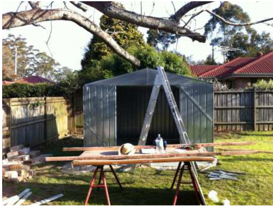
Figure 32.: Tuesday afternoon 3:49pm – roof panels installed!
