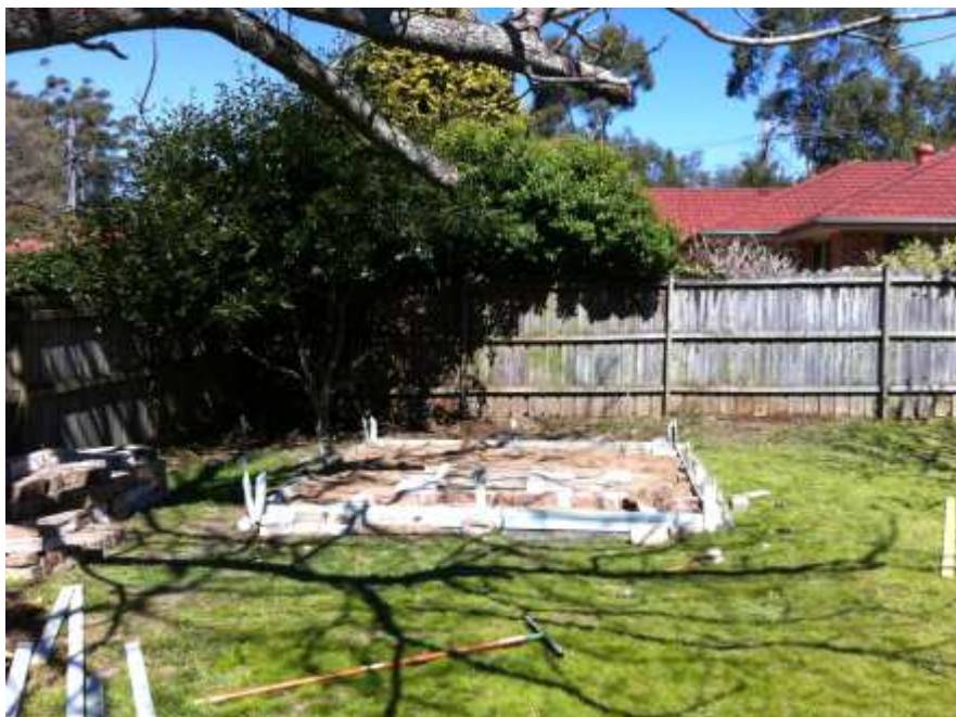
Figure 20.: Sunday afternoon 12:09pm – progressing with the brick pad
