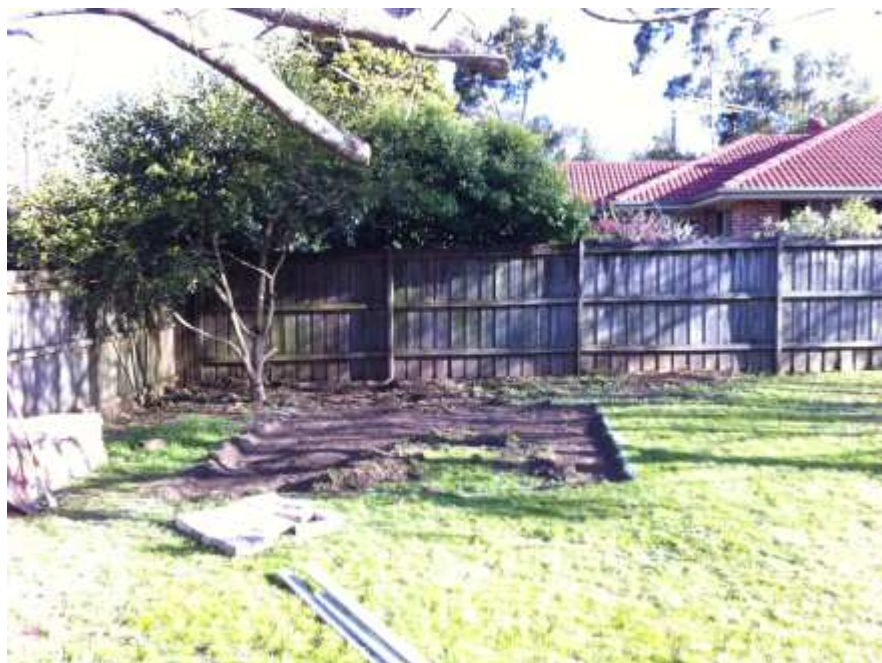
Figure 9.: Friday afternoon 3:56pm – making progress with the digging
