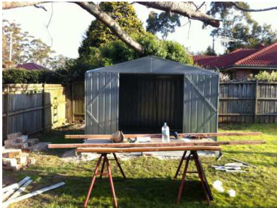
Figure 33.: Tuesday afternoon 4:25pm – internal roof struts installed
