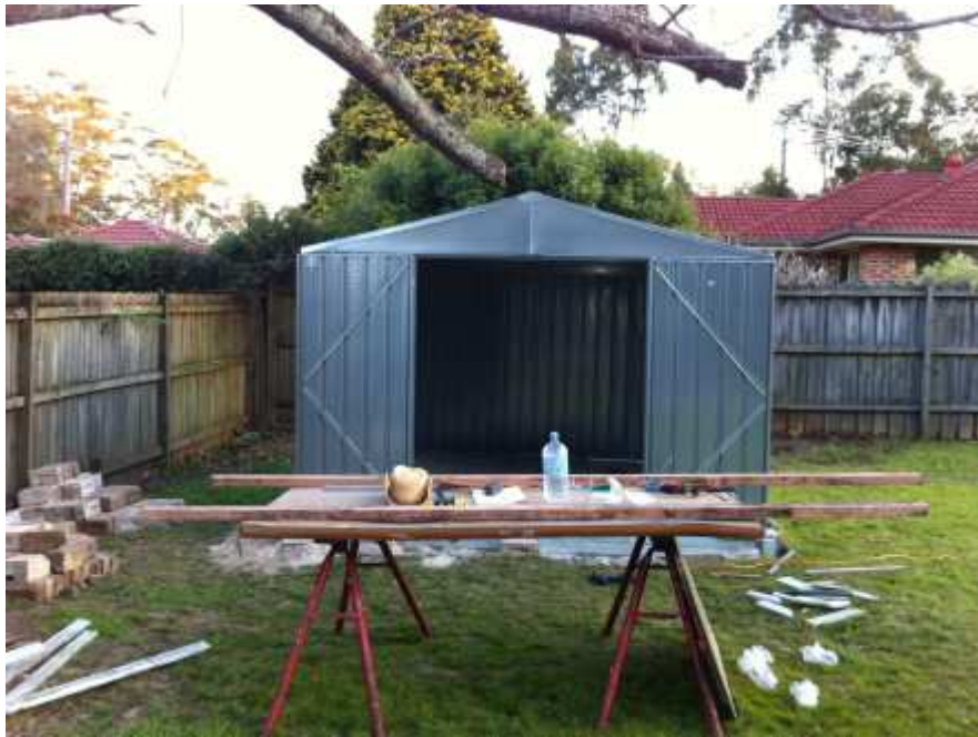
Figure 34.: Tuesday afternoon 5:13pm – roof secure, gable caps on
