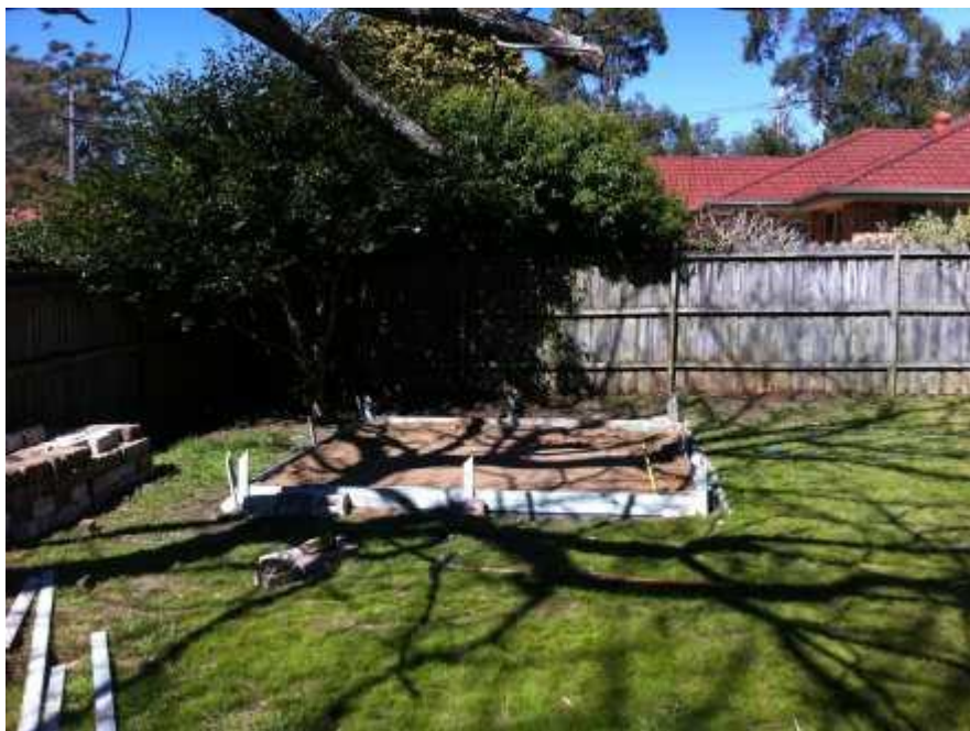
Figure 18.: Sunday morning 10:18am – levelling up the sand bed
